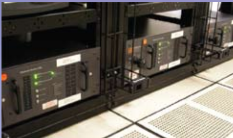
TwinSource RMSTSs Installation in Racks
